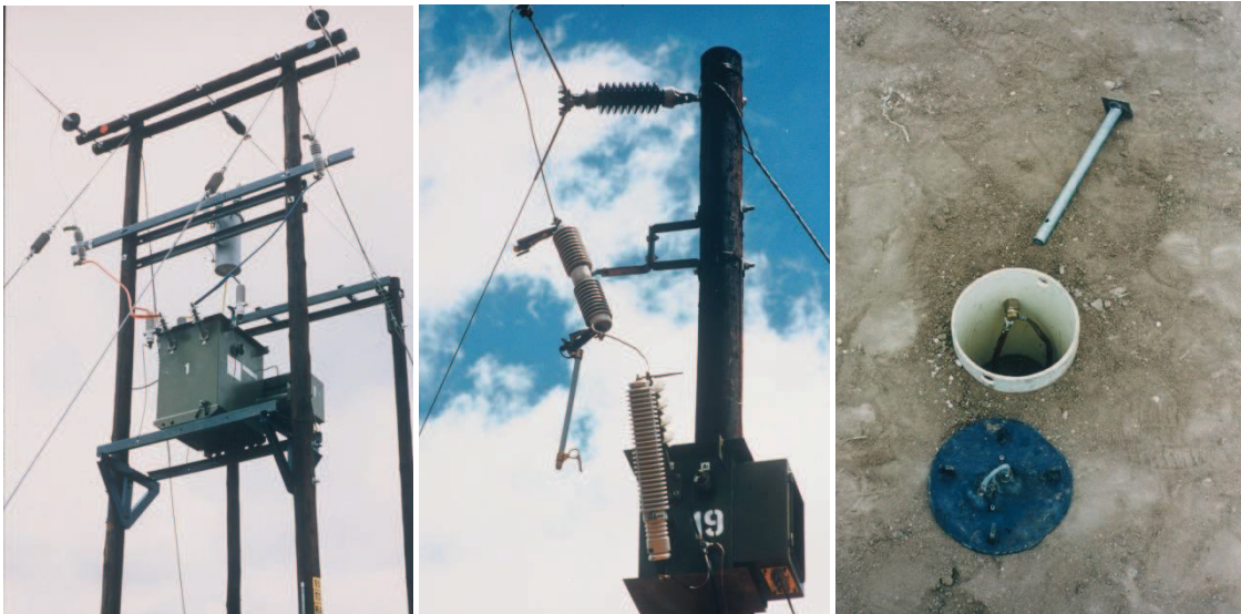
FIGURE 22 - These photographs from the first Botswana SWER system illustrate the simplicity of SWER systems: an isolating transformer with input from two phases, a load transformer connected to the line and the top of the earthing electrode that carries the current into the ground.
